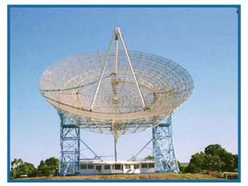
was erected, it was the third-largest antenna of its kind in the world. It has unique capabilities in frequency coverage, tracking speed, extracting weak signals from noise, and transmitting range. At first it was used principally to beam signals to a number of very distant spacecraft probing the solar wind in a joint SRI/Stanford project.
