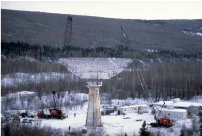
Figure 4. The removal of the reflector and torque tube from the gun mount, preparatory for shipping the ISR system to Greenland (photo by C. Heinselman).
