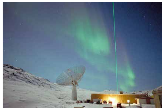
Figure 5. The Sondrestrom Upper Atmospheric Research Facility, showing the 32-m fully steerable parabolic dish, Rayleigh lidar beam, and aurora on a moonlit night (photo by C. Heinselman).
