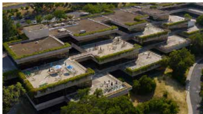
SRI’s PARC campus – where the PARC forum resumed in April 2024.
