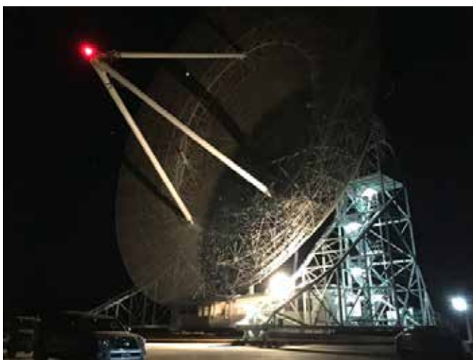
The Dish as used the night of the MarCO test.
